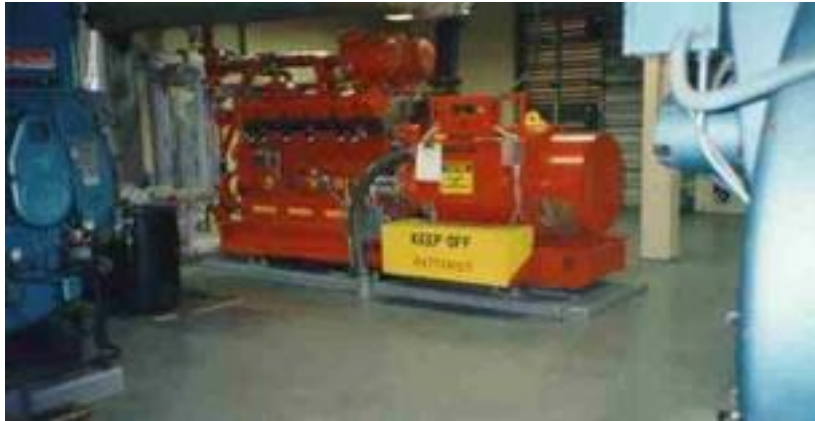
Photo 3. A Model for Electricity Generator Unit from Methane Gas in Wastewater Treatment Plant (Reference 9)
