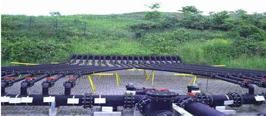
Photo 1. A Model for Horizontal Collection of Gas Pipes in a Landfill (Reference 10)
