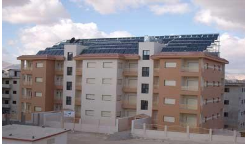
Figure 8: Qudsaya Youth Building Pilot Project in Damascus, Syria
