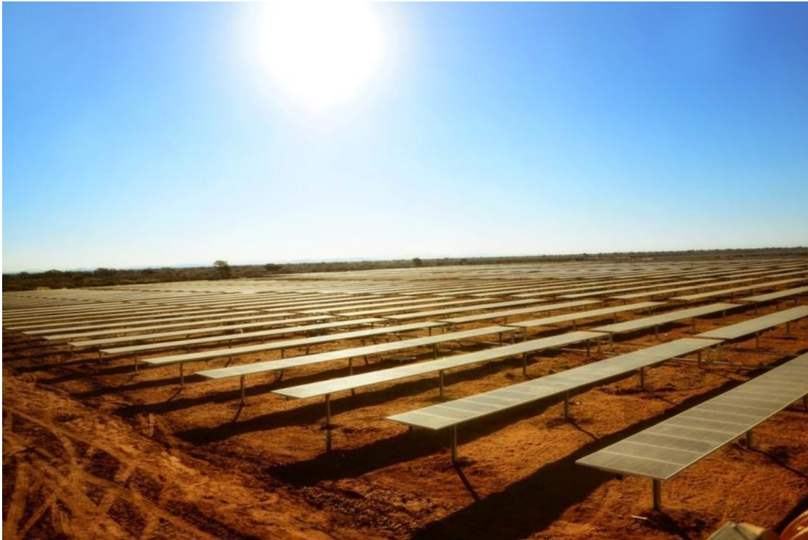
Figure 16 Off-site photovoltaic plant. Source: Acciona Ingeniería
