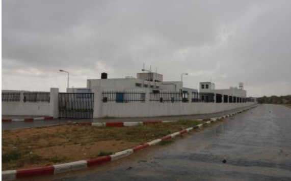
Figure 6 Northern part of the project site: STLV Sea Water Desalination Plant (6000 m 3 /d) by PWA with support from UNICEF and EU. Source: Acciona Ingeniería
