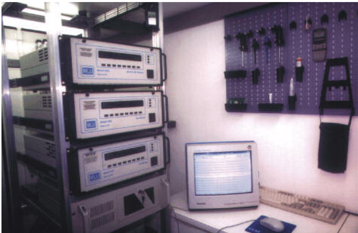
Figure 15: Automatic analysers and the control computer in the Mobile Unit.
